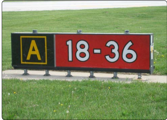
Figure 1-20. Runway holding position sign at a location other than the takeoff end of Runway 18-36 with colocated Taxiway Alpha location sign.
