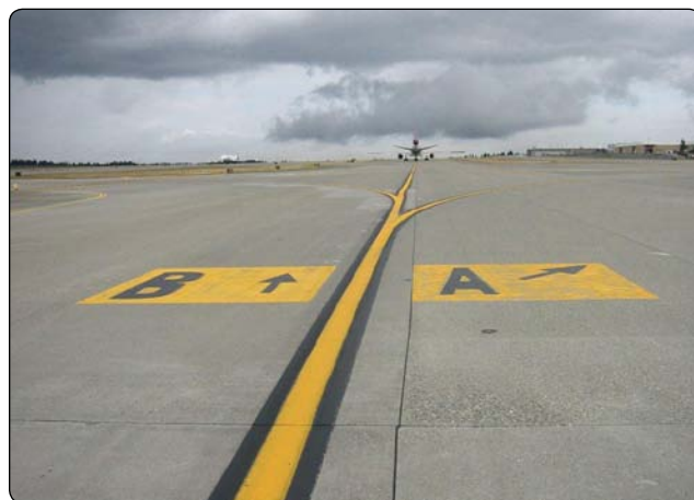
Figure 1-32. Surface painted taxiway direction signs.
